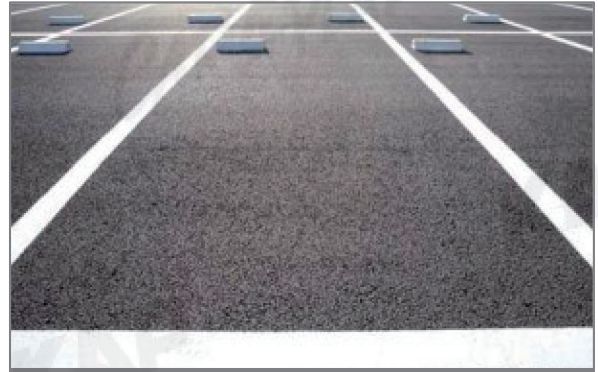
Parking Line OFF Screen
